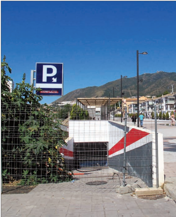
Pueblosol, a finished car park not being used.
