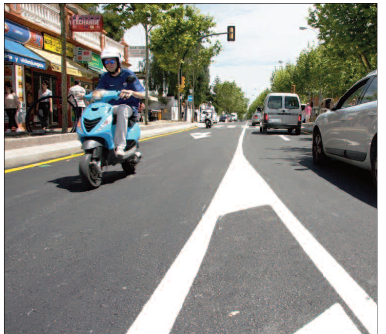
The ugly construction barriers are a thing of the past.
